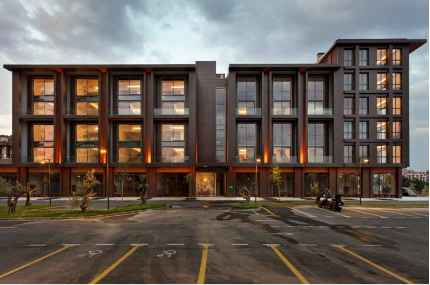
Private residence, Bursa (Turkey) Ventilated façade: Iron Corten Designed by: Işıl Gençođlu-Süleyman Taşar Image: Burak Teoman
