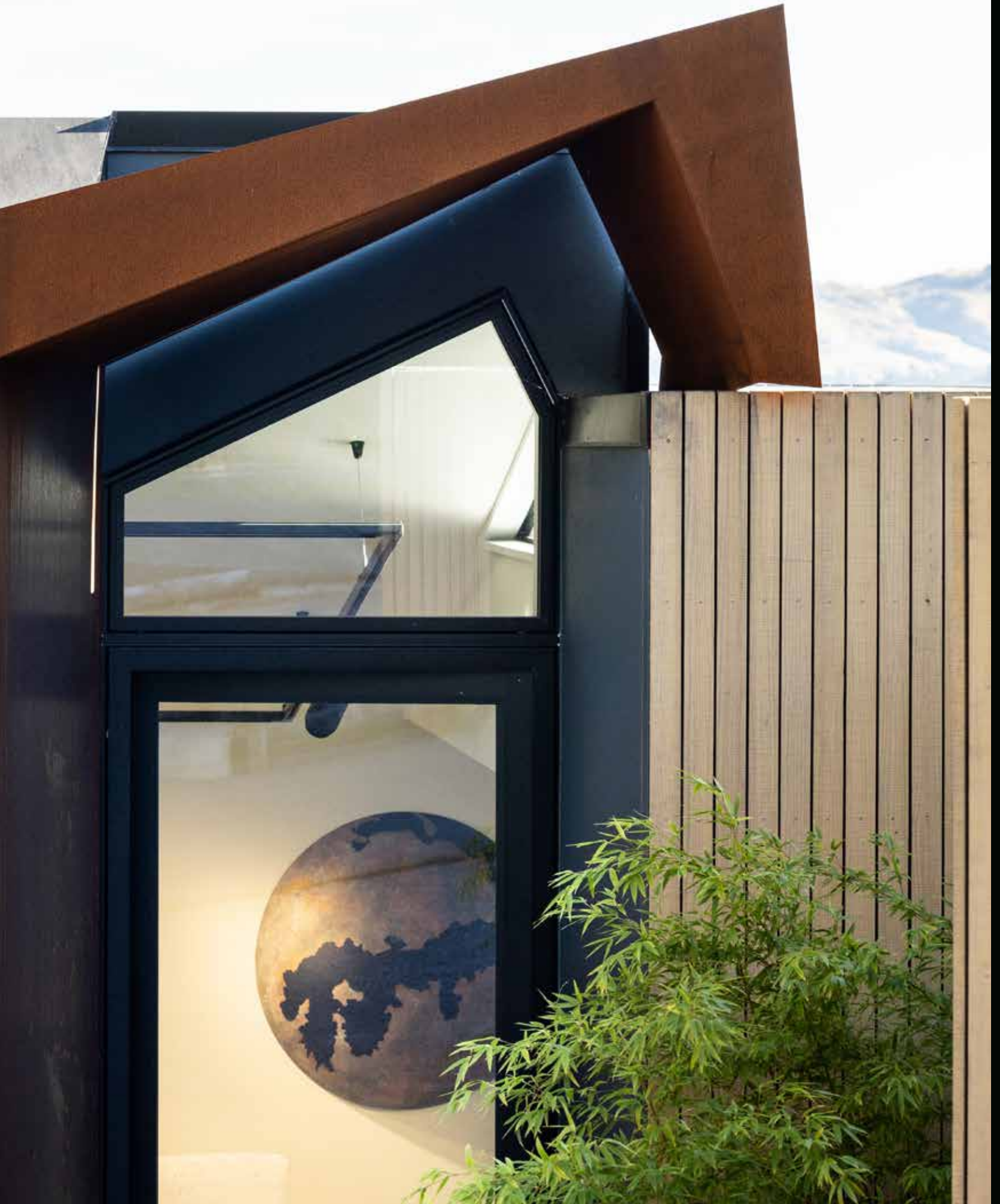
Private residence, Christchurch (New Zealand) Ventilated façade: Zaha Stone and Basalt Black Designed by: MC Architecture Studio Ltd Image: Clinton Lloyd
